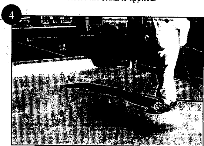
Foam Application: The closed-cell spray polyurethane foam is applied over the existing roof.
