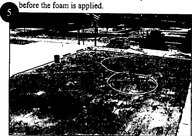
Before/Foam & Base Coat: Foam is sprayed over prepared roof, then acrylic base coat is applied over the foam.
